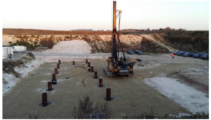
Figure 45. ALPACA LD piling operations at St Nicholas at Wade; November 2017.
