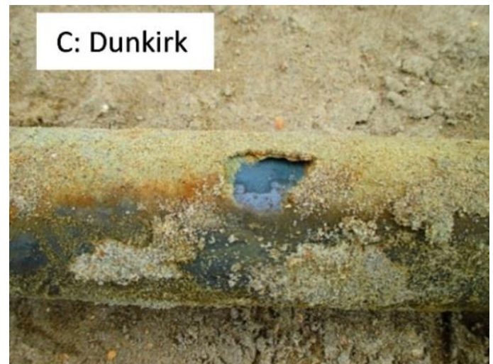
Figure 56. Open-ended mild steel 50mm OD micro-pile retrieved 2 years after driving above the water table, note \approx 1 mm thick adhered sand grain zone bonded with corrosion product.
