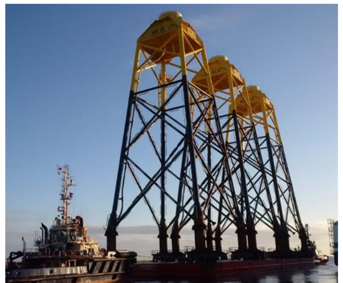
Figure 43. Three OWT jacket structures in transit to Wiking; photograph courtesy of Scottish Power Renewables.
